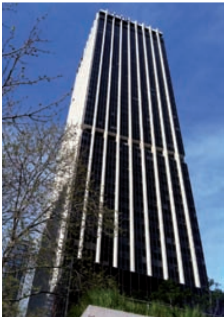
Bridge Street Tower
