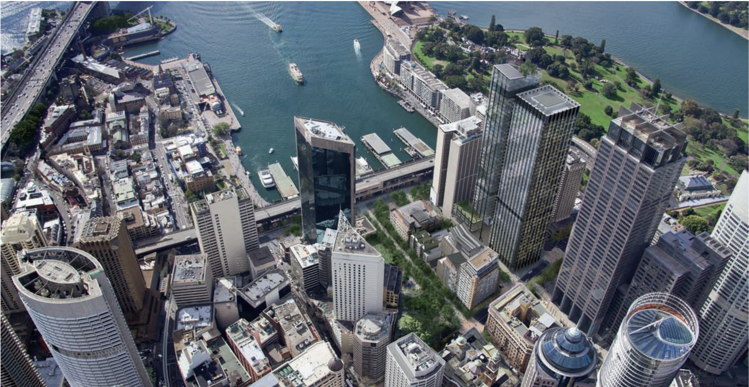
Bridge and Alfred Street Block
